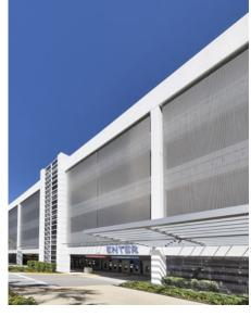
The project team worked with GKD to come up with something attractive and durable that involved 17,678 square feet of GKD's Omega 1520, embodied in 22 panels that are approximately 39' tall by 20' wide. The unique installation used 904L cabling in conjunction with T316L stainless rods, providing superior resistance to oxidation.
